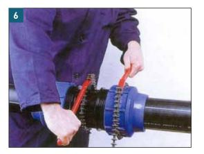
Tighten the nut manually: then tighten it further with a special wrench. It is not necessary for the blue not to be in contact with the external stop of the body.
