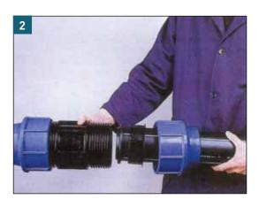
Disassemble all the fitting components. Make the nut, the black bush and the O-ring slide onto the pipe setting them near the pipe's end. Do not use the white clamping ring at this stage. It is helpful to lubricate the pipe's end and the O-ring with a suitable lubricant that does not affect the drinking water properties.
