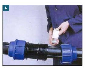
Unscrew the nut and put the white clamping ring onto the pipe.
