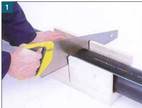
1 Cut the pipe squarely using special pipe cutting tools or circular or band saw. it would be better to use a sawing guide to obtain a square cut.
