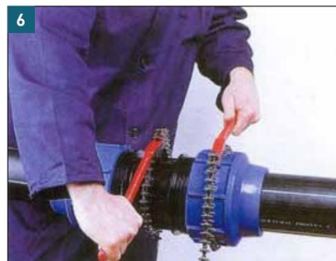
6 Tighten the nut manually: then tighten it further with a special wrench. It is not necessary for the blue nut to be in contact with the external stop of the body.
